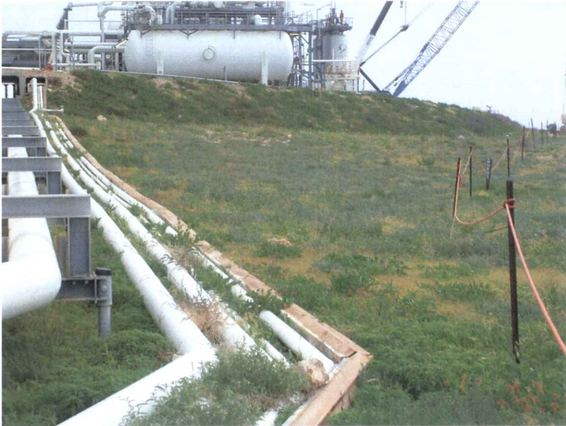
Photo 1. Vegetation under pipelines and cable trays.
