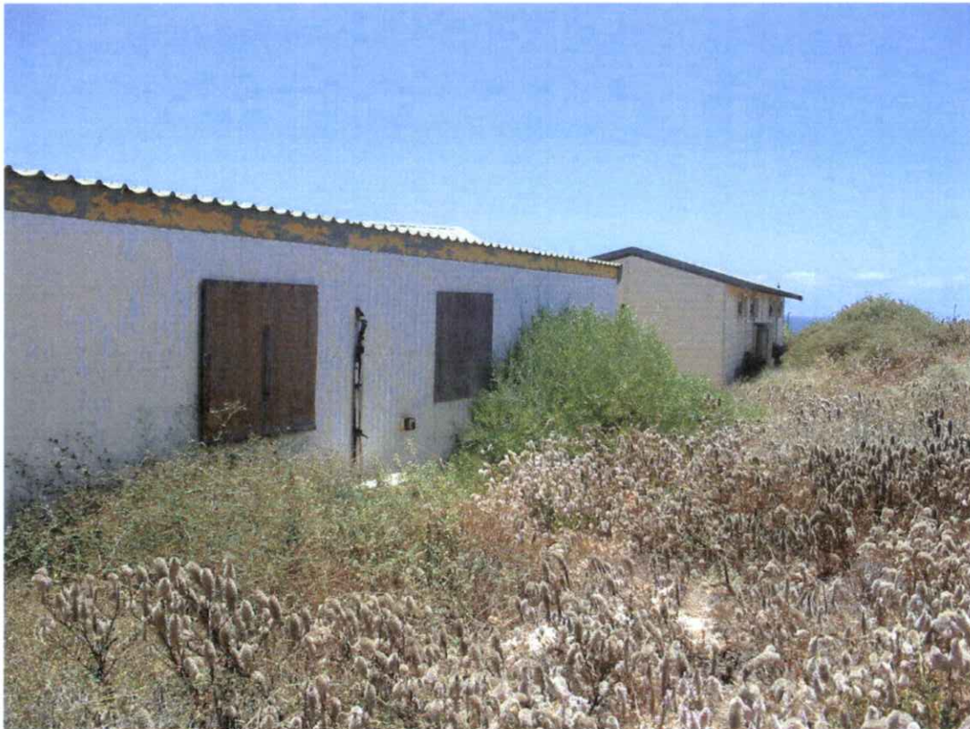
Photo 2. Vegetation around base of accommodation units.
